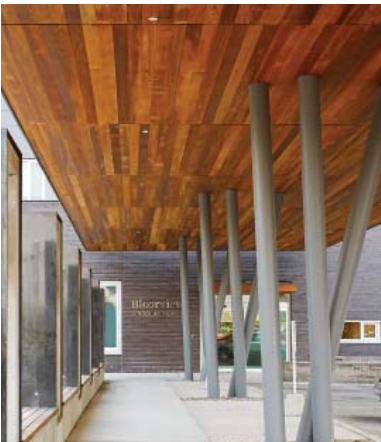
entrance canopy at school
