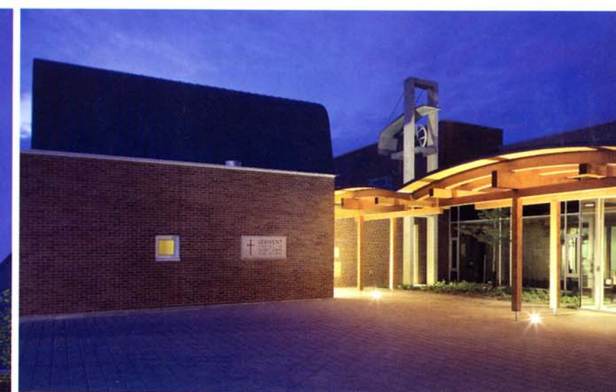
Previous page top, left and above: The complex consists of a two-storey elemental brick volume with a random pattern of vertical window openings. The exceptions to this are the chapel and the timber-frame entrance canopy flanked by a concrete bell tower, elements whose distinct forms give them particular significance in contrast to the simplicity of the brick wall.
